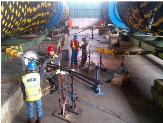
Installing Connectors on Power Cables (Credit: FORCE)
