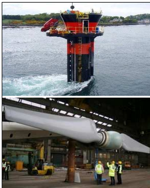
Figure 7: Example of a tidal stream energy conversion device; the Marine Current Turbines SeaGen device. (Source: Marine Current Turbines). www.marineturbines.com
