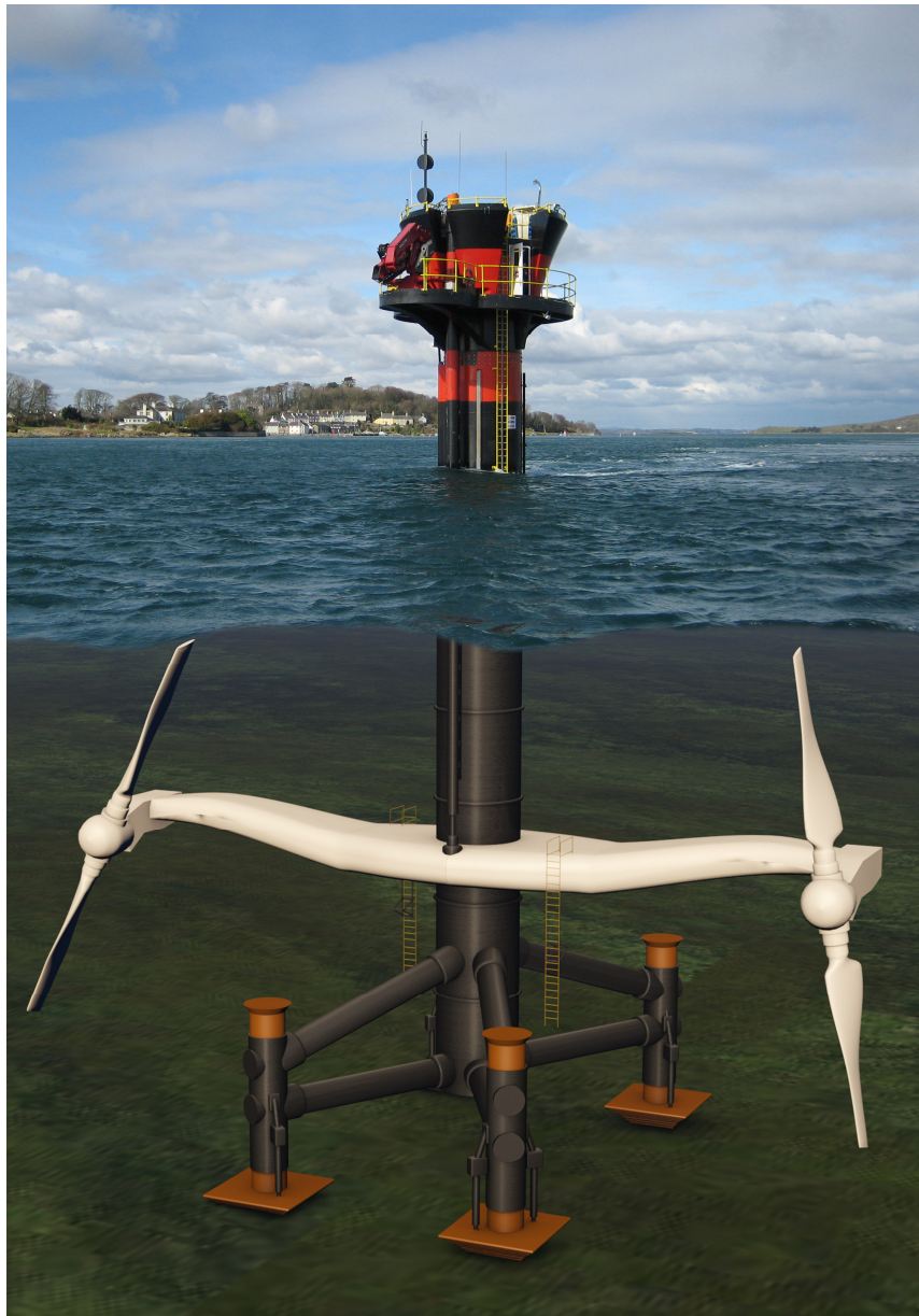
Figure 1.1: The SeaGen turbine, Strangford Lough, Northern Ireland.
