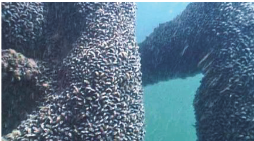
Figure 38: Colonisation by mussels ( Mytilus Echilij ) on protective structures of the Horn Rev offshore wind farm, Denmark
